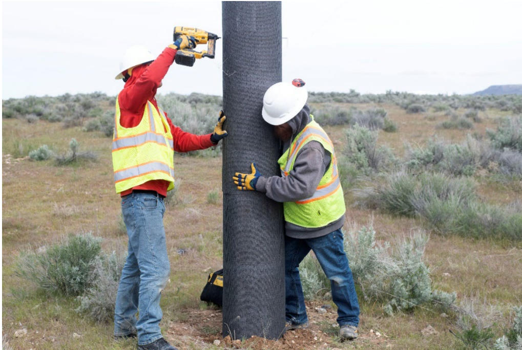
Figure 1 A field team installs a mesh wrap on a wood pole in 2022
